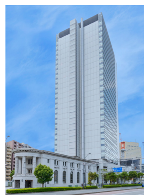
Yokohama i-land Tower
