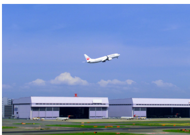
IIF Haneda Airport Maintenance Center
